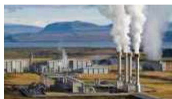
Fig 8.11(b) Geothermal power plant
