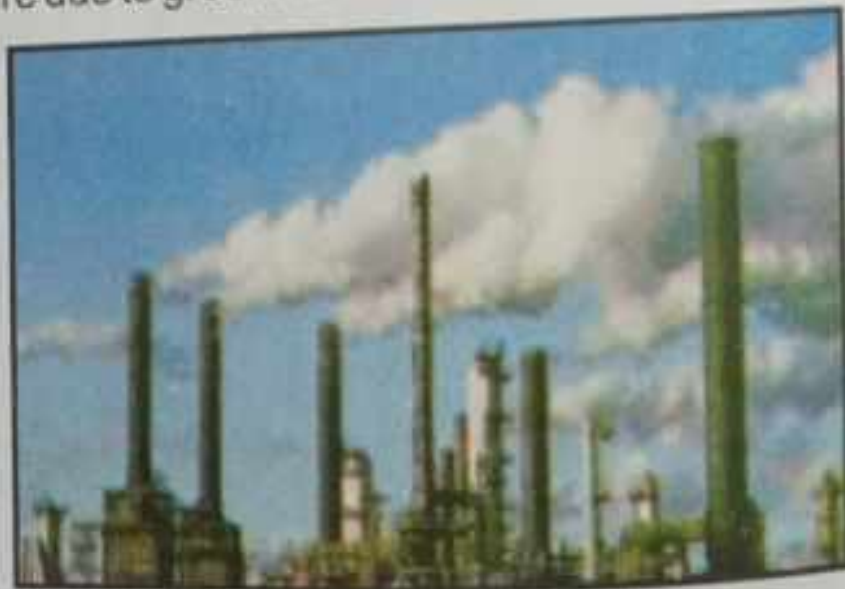
Fig: 5.12 Thermal pollution emitting from chimneys.
