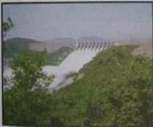
Fig: 4.4 Terhola dam because of which the reservoir has lost the storage capacity to a reasonable level and now the dam is left with two-third capacity to store water.
