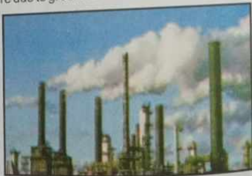
Fig: 5.12 Thermal pollution emitting from chimneys.
