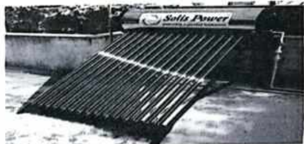
Fig. 6.8: Solar water heater
