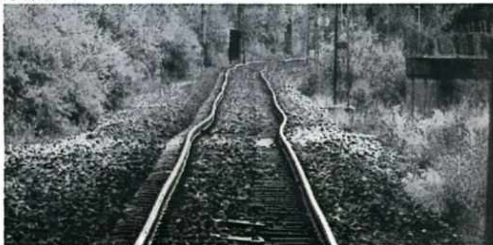
Fig. 10.8: Expansion in railway track
