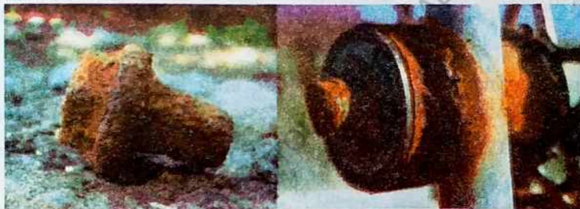
Figure 7.7 Rust in Iron
