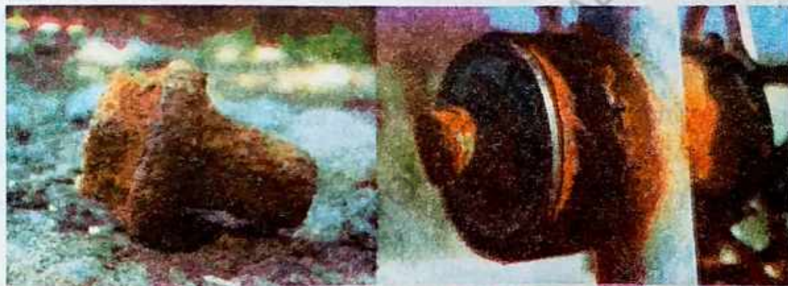
Figure 7.7 Rust in Iron
