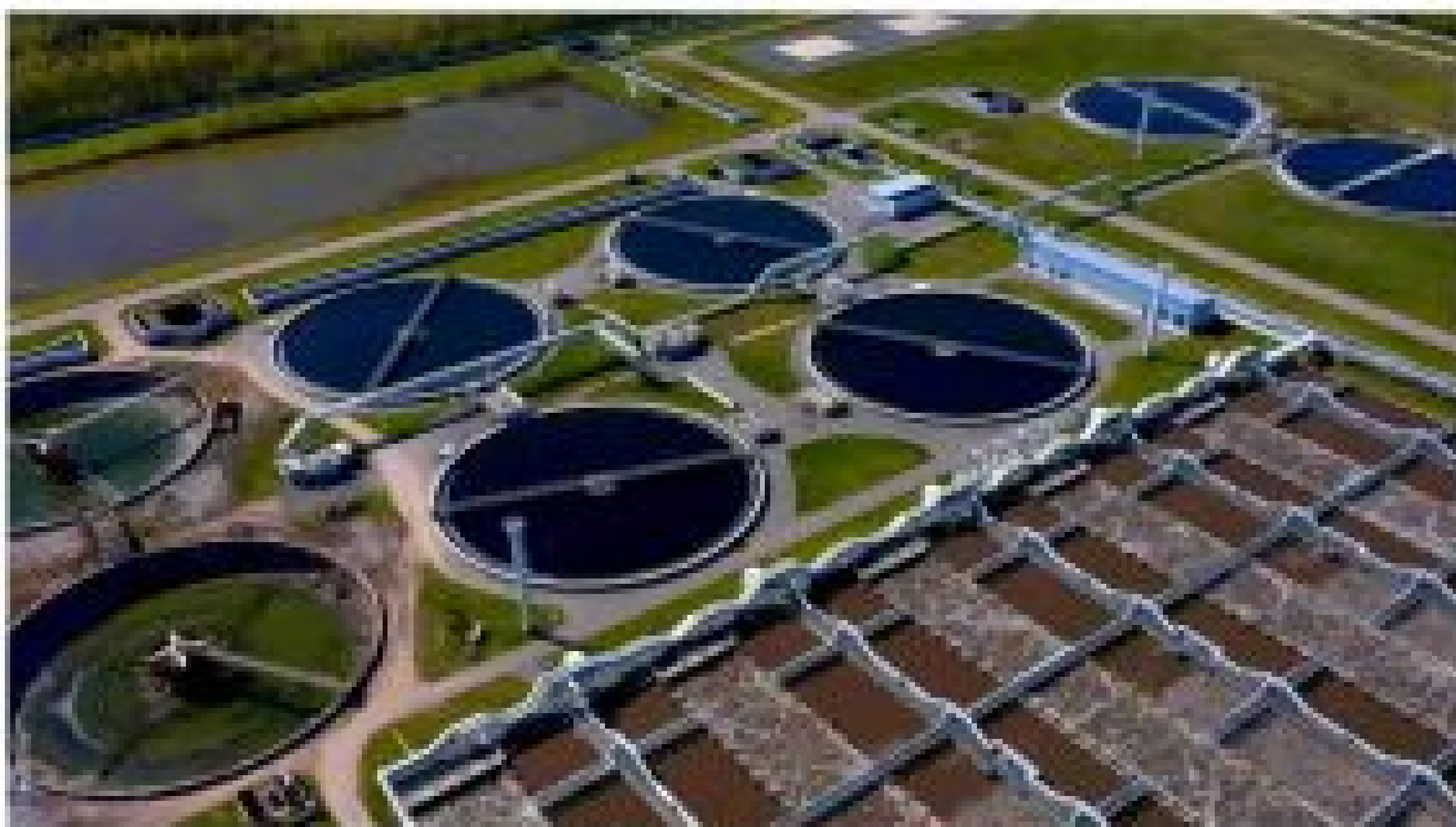
Fig. 27.7 Sewage treatment plant
